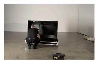
4. Remove the transport bolts in each side to unlock the OLED Housing from the flight case. Use the wrench and Umbraco key size 8 for this.
