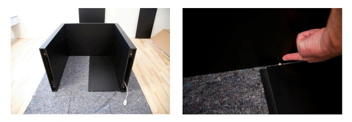
If you find it difficult to get the pins into the holes, you can attach the self-adhesive felt pads on the back side of the Back-Wall part to get the perfect height. Remove them again after assembly.
